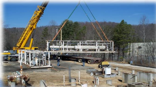
Equipment Setting and Rigging
