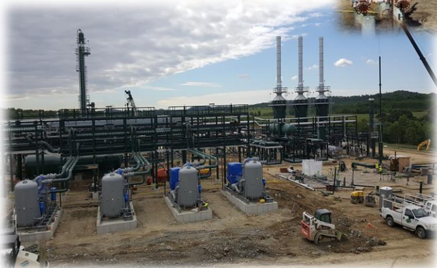
Natural Gas Piping Installation
