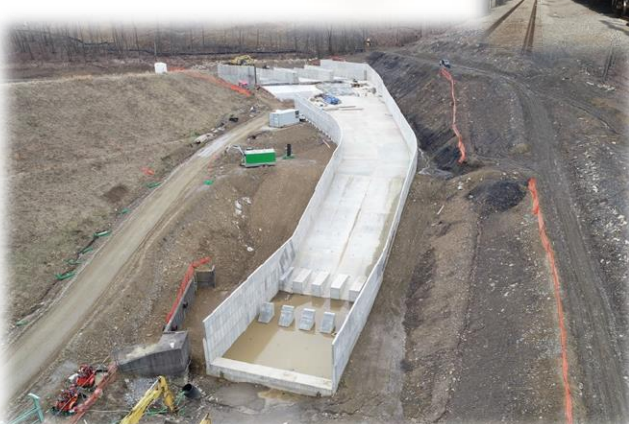
Dam and Spillway Construction
