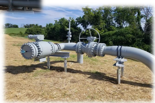
Helical Piles and Pipe Coating
